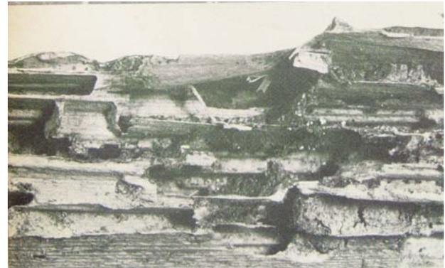
**Termite damage in structural timber**
